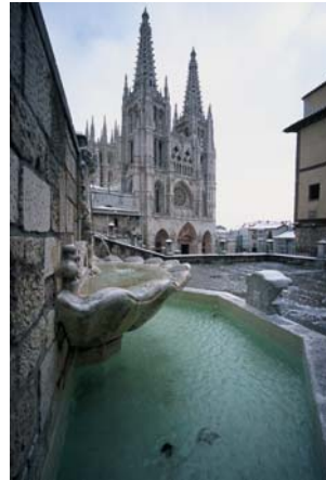
Renovation of the Burgos cathedral façade in Spain
